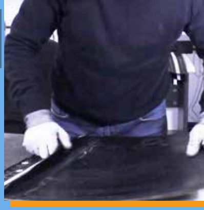
19) Place the second end of the belt into the splice, make sure it butts up against the opposite side that was previously marked and align the two sides of the belt using the bias. The two ends of the belt should connect.
